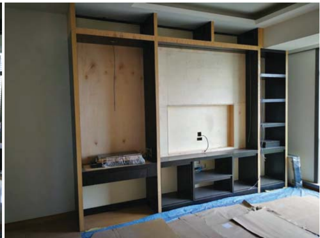
type A : work progress
